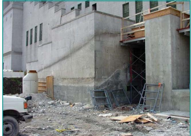
PROVOTON foam concrete was used to backfill and support original exterior stairway.
