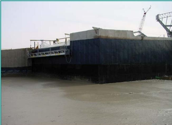
PROVOTON foam concrete being placed against north garage walls.
