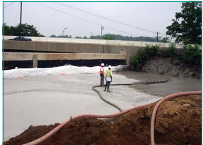
Filling up the north side of the Woodrow Wilson bridge abutment.
