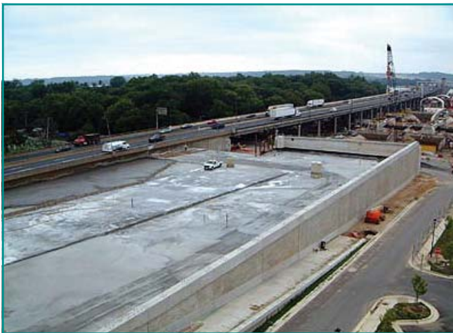
The Virginia abutment backfill utilized 60,000 cy of PROVOTON foam concrete.
