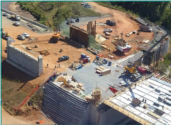
Finished backfill of one of the Maryland side connector bridge abutments.
