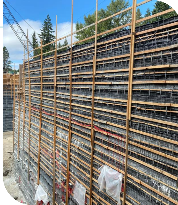
Overpass Abutment Backfill
